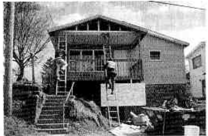
Nazareth Farm volunteers attach siding to the McKinney's new Habitat house in West Union. photo/Larry Spollen
